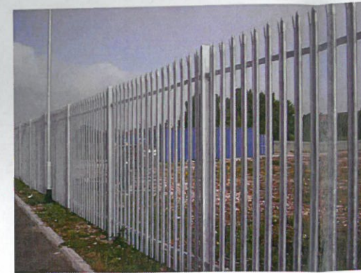
IMAGE SHOWING TYPICAL FENCE ARRANGEMENT
